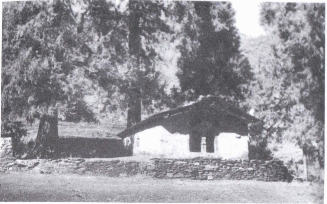
Fig. 4: Shrine (thān) at Jajallo in Bajhāng, view from the south.
